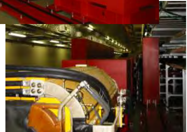
New absorbers and wall-type shields in ring-collimator area
