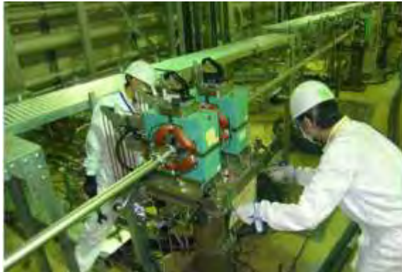
Alignment of L3BT electromagnets
