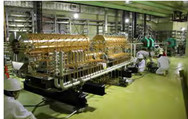
Installation of ACS in Tunnel
