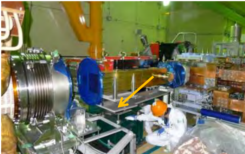
Installation of New Collimator
