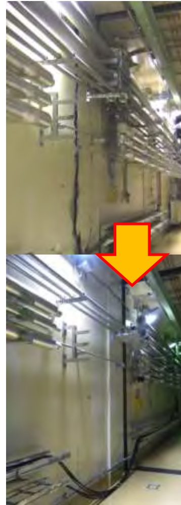
Restoration work of an expansion joint in 3NBT tunnel was completed.
