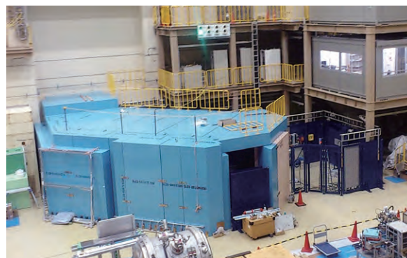
Fig. 7. Part of the S-Line completed to the S1 Area (the first of four planned branches).
