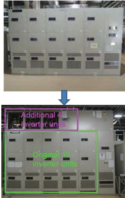
Fig. 9. Reinforcement of the anode power supply system.
