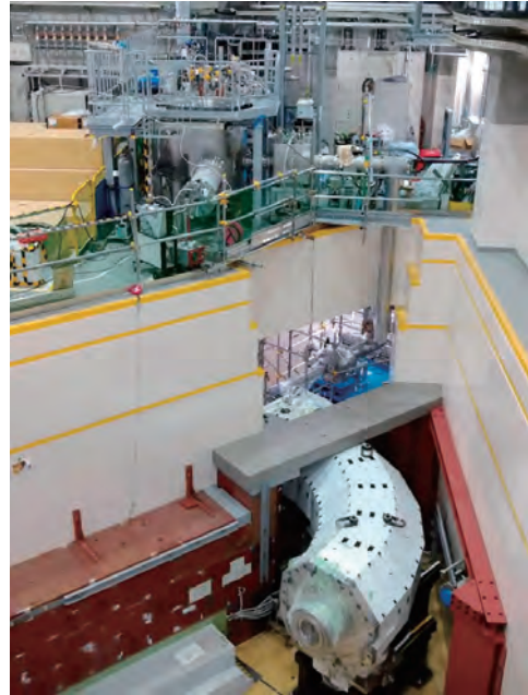
Fig. 8. MTS cooling system
