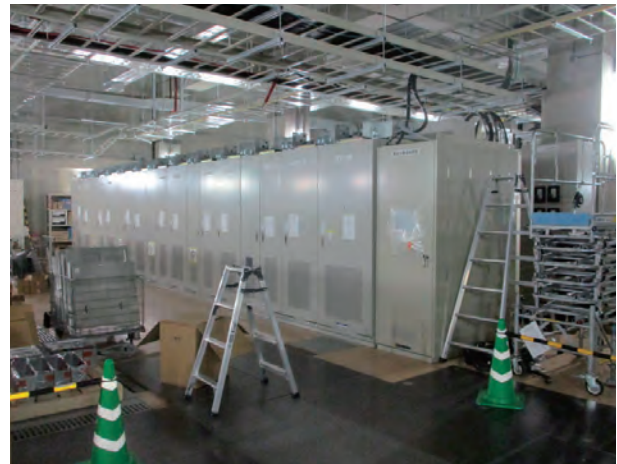
Fig. 2. New magnet power supply for a quadrupole family of QDN.
