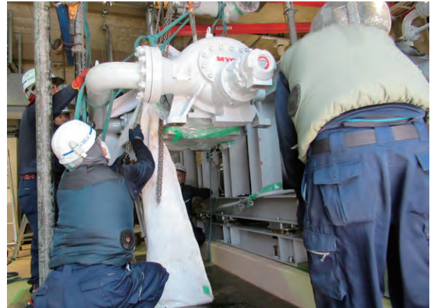
Fig. 4. Uninstalled LHe compressor.
