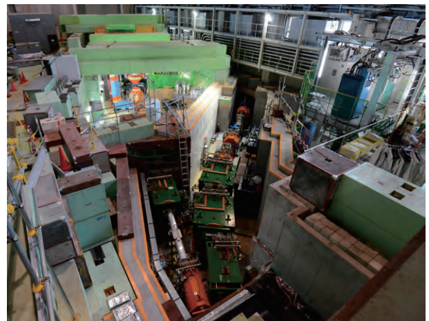
Fig. 1. Photograph of the branch point of B (to up direction in the figure) and C (to right up direction) lines in Hadron Hall taken before closing the shielding structure.
